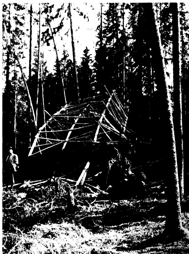
Fig. 2. — Scaffolding and plus tree have blown down.
