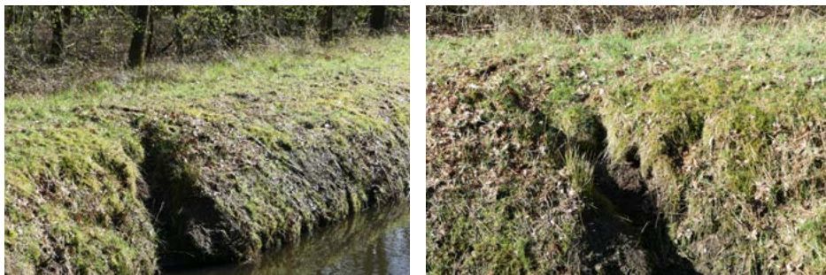
Figure 1: Strong burrowing activity by rodents in the dam of a fish pond, photos: © Thünen Institute / Vincent Lugert.
